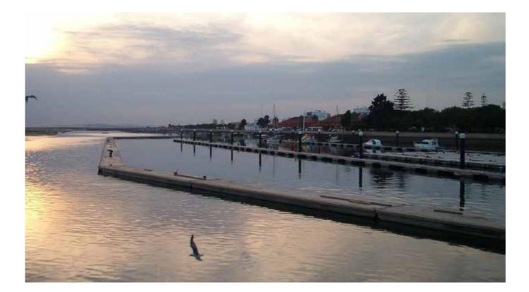
The QMF (Floating Wave Attenuator) range consists of robust, resistant and safe pontoons made of reinforced concrete with an expanded polystyrene core. Its geometry, layout, construction method and type of connections make its primary use as a wave attenuator in the protection of bays and ports.
