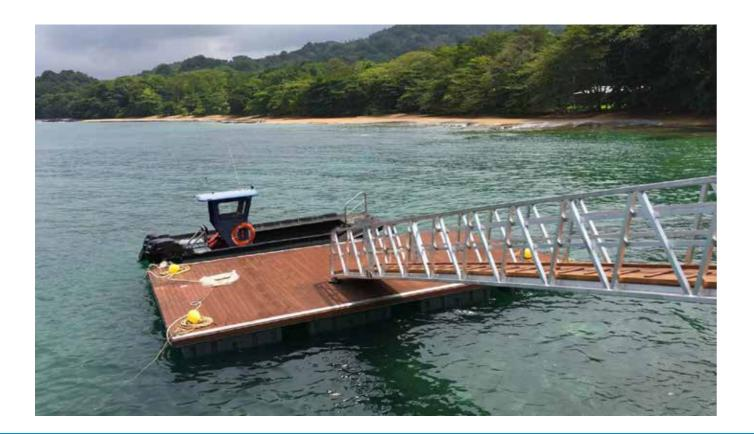
The Faro and Faro+ systems consist of floating pontoons with a special aluminum alloy profile structure composed of modular units.
