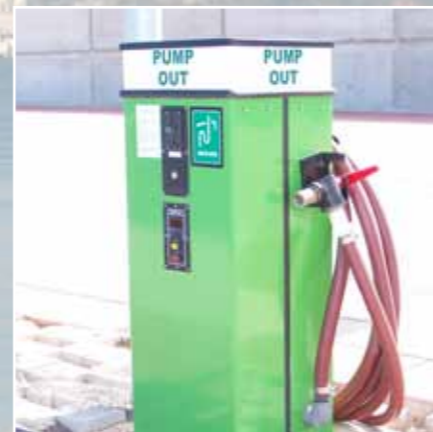
Sanitation Pump-Out Pedestals
