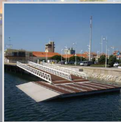
Access Bridges and Ramps
